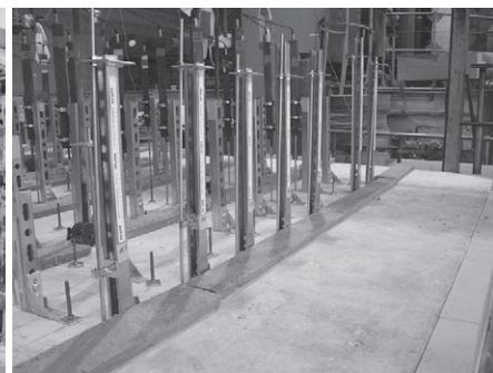
Fig. 2: Measurement system for recording the load behavior of the systems in the furnace
